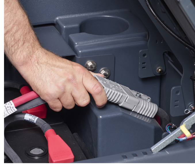
3. Check battery cables are well connected together
